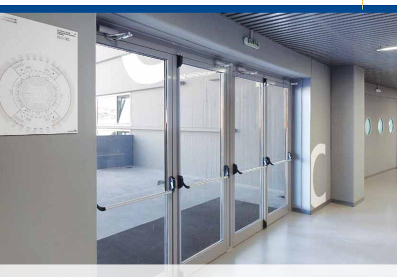
GEZE TS 1500 / TS 2000 / TS SYSTEM 4000 OVERHEAD DOOR CLOSERS WITH LINK ARM
